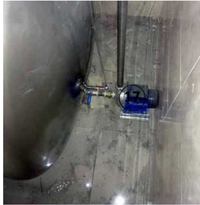
16. The accumulated tank water in the tank is pumped into the oil water tank with the pump.
